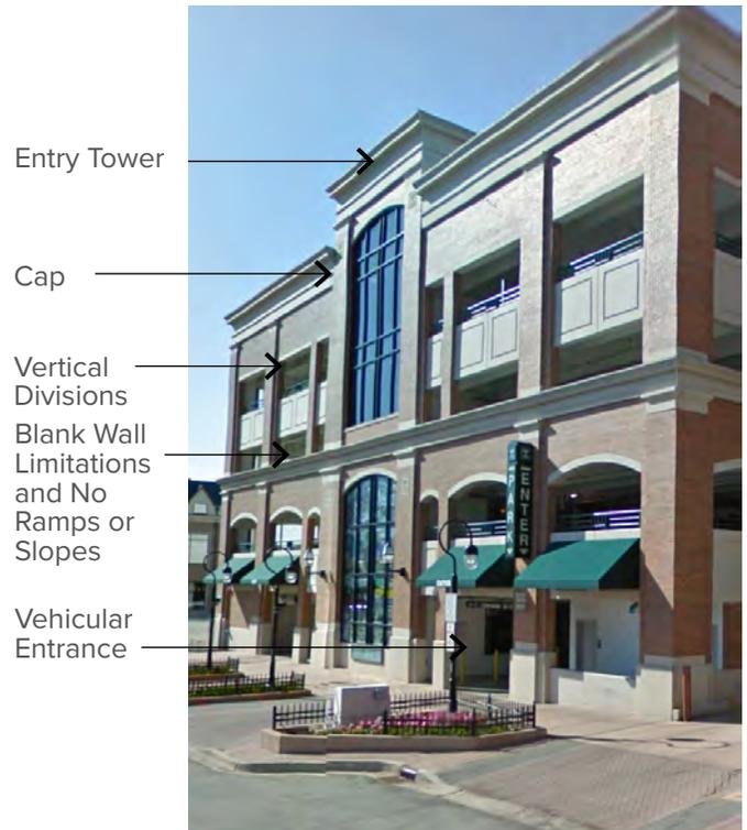
**Figure 5-K.** Example of Parking Structure Facade on a Street
